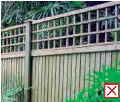
Timber fencing with trellis addressing the public realm will not be acceptable, except as a temporary measure to phasing boundaries.
