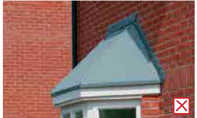
Bay windows and dormers with poorly designed GRP details will not be acceptable.
