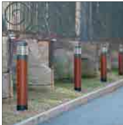
Low level, timber/metal lighting bollard (if required to non-adoptable pedestrian paths only)
