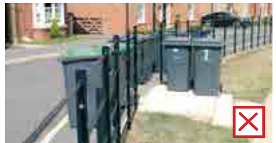
Bin collection point for 3 or more dwellings should never be placed along a public open space or a primary street.
