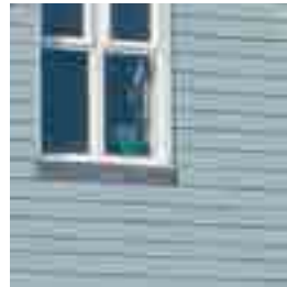
Stained or painted weatherboarding various colours
