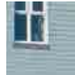
Stained or painted weatherboarding various colours
