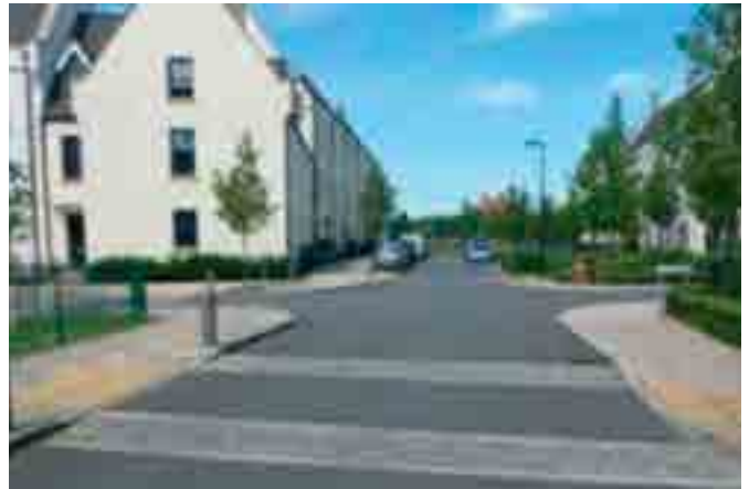
Raised table crossings act as speed restraints and also assist frame and wheelchair users and people pushing buggies (Images courtesy of WSP | Parsons Brinckerhoff)
