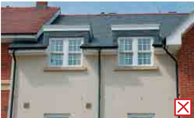
In order to reduce unnecessary clutter of rainwater pipes, excessive numbers of dormer windows in closed proximity which break the eaves line will not be permitted.
