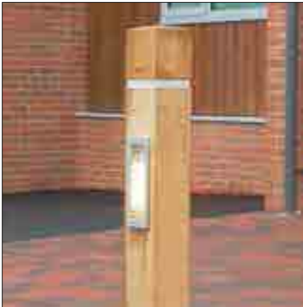
Low level, timber lighting bollard (if required to non-adoptable pedestrian paths only)
