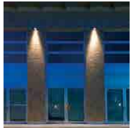
Accent lighting to façades
